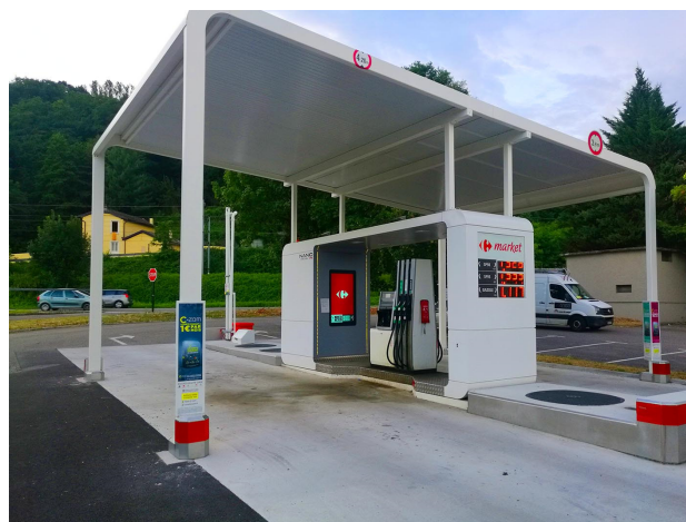
Picture 4: a temporary / small plug&play gasoline station, Bourgoin Jallieu, France, 2017
