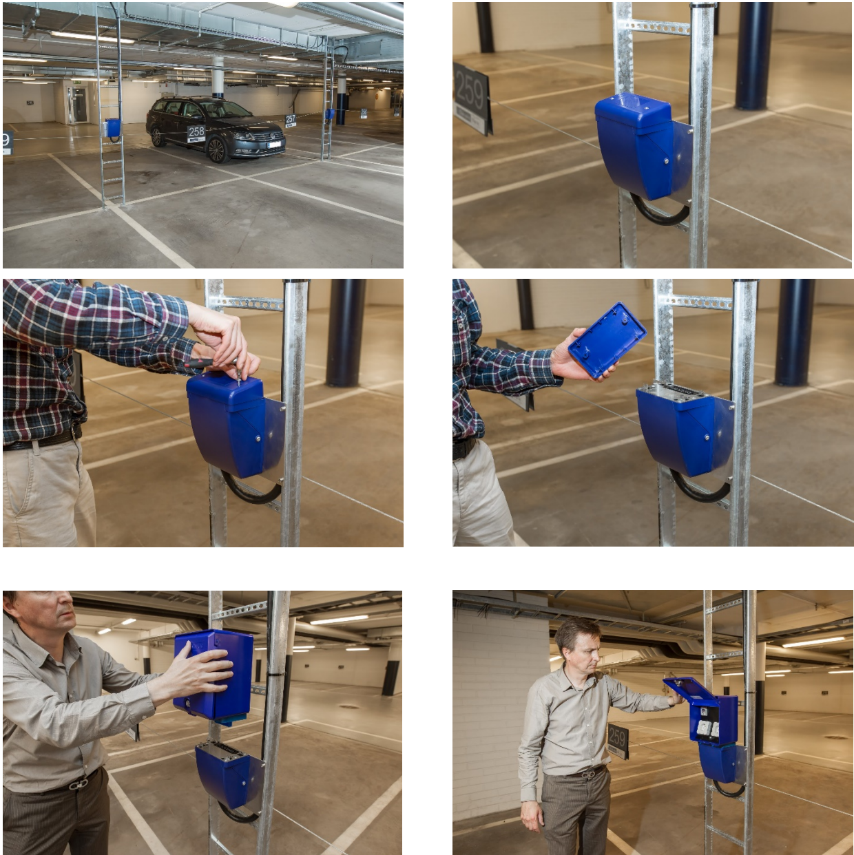
Figure 1: Installation of Charging unit to a quick connector
