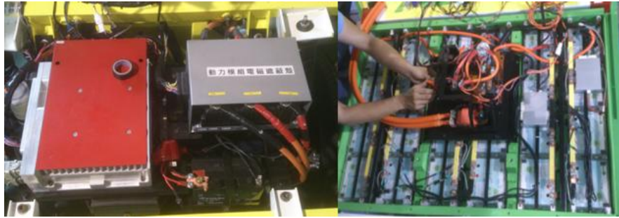
Fig. 7: Actual installation of the shielding shell
