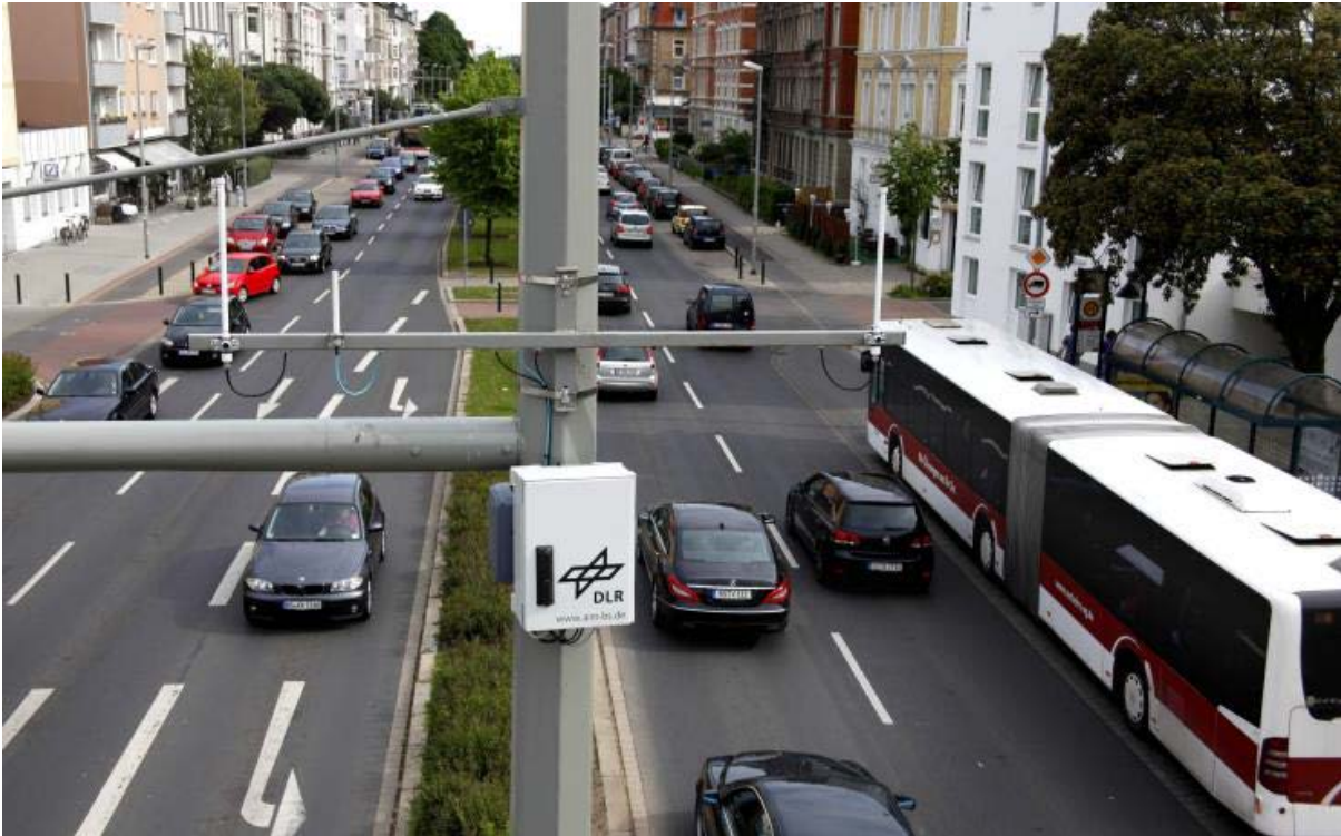
Figure5: Transmitters and Receivers for vehicle-to-infrastructure communication (V2X)
