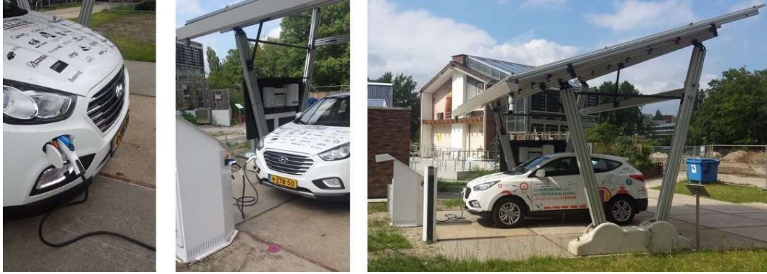
Figure 1: Experimental Fuel Cell Electric Vehicle-to-Grid (FCEV2G) 10kW set-up at Delft University of Technology.
