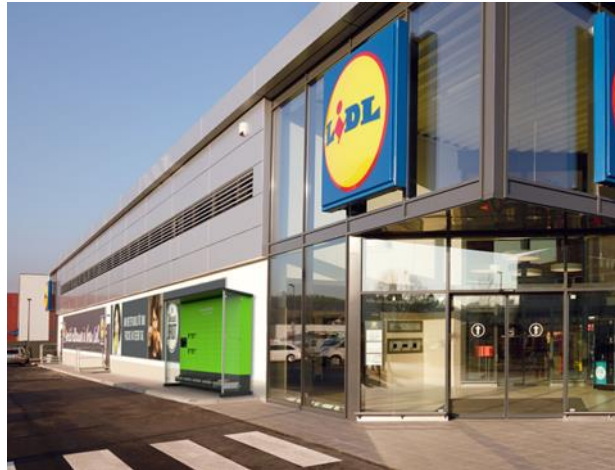
Figure 8: GreenPack swapping station at a supermarket
