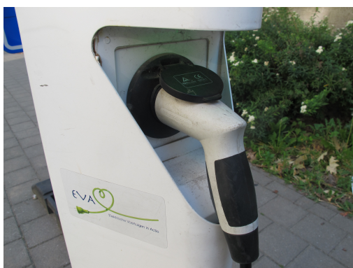
Figure 4: Type2 plug at charging post
