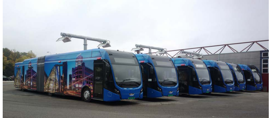
Depot charging at Eindhoven bus depot
