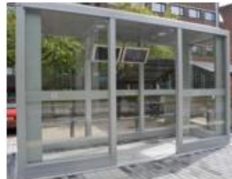
Bus stop with sound-deadening technology
