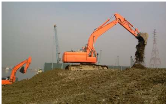
Figure 15: Prototype hybrid excavator
